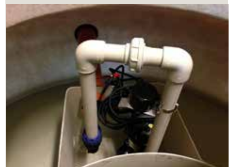
Pumpepakke for BAGA slamavskiller.
